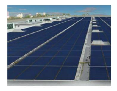
The panels employ cylindrical modules which capture sunlight across the photovoltaic surface and convert direct, diffused and reflected sunlight into electricity. The panels achieve effective energy generation when mounted horizontally and spaced significantly closer together than conventional panels on a typical rooftop, thereby enabling greater rooftop coverage and enhanced energy production.
